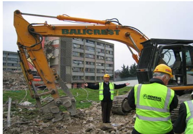
Former estate on Tanner Street undergoing demolition
