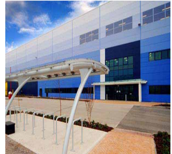
Voltac building, Dagenham Dock
