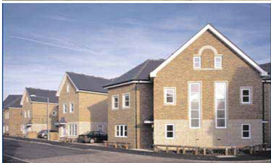
Charlecote Road, Dagenham
